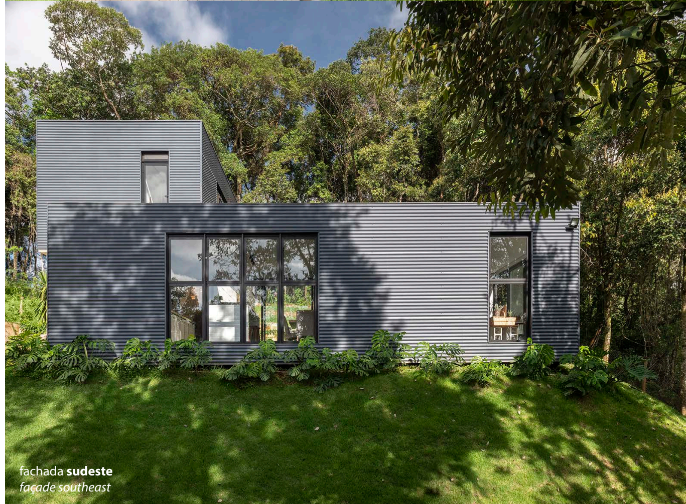
fachada sudeste façade southeast
